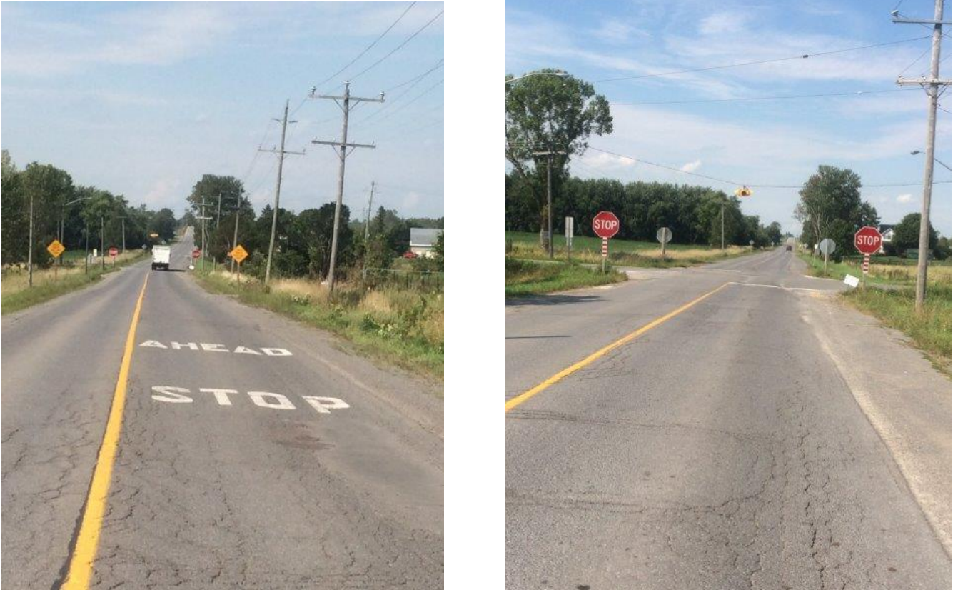
Figure 8-2. Intersection of County Road 1 and County Road 10 from South
